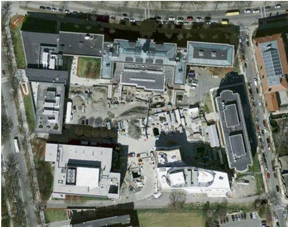
Figure 31 Aerial Image of Initial Construction Site
